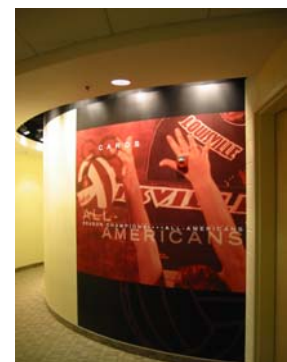
Notice where the fire alarm pull station is?
