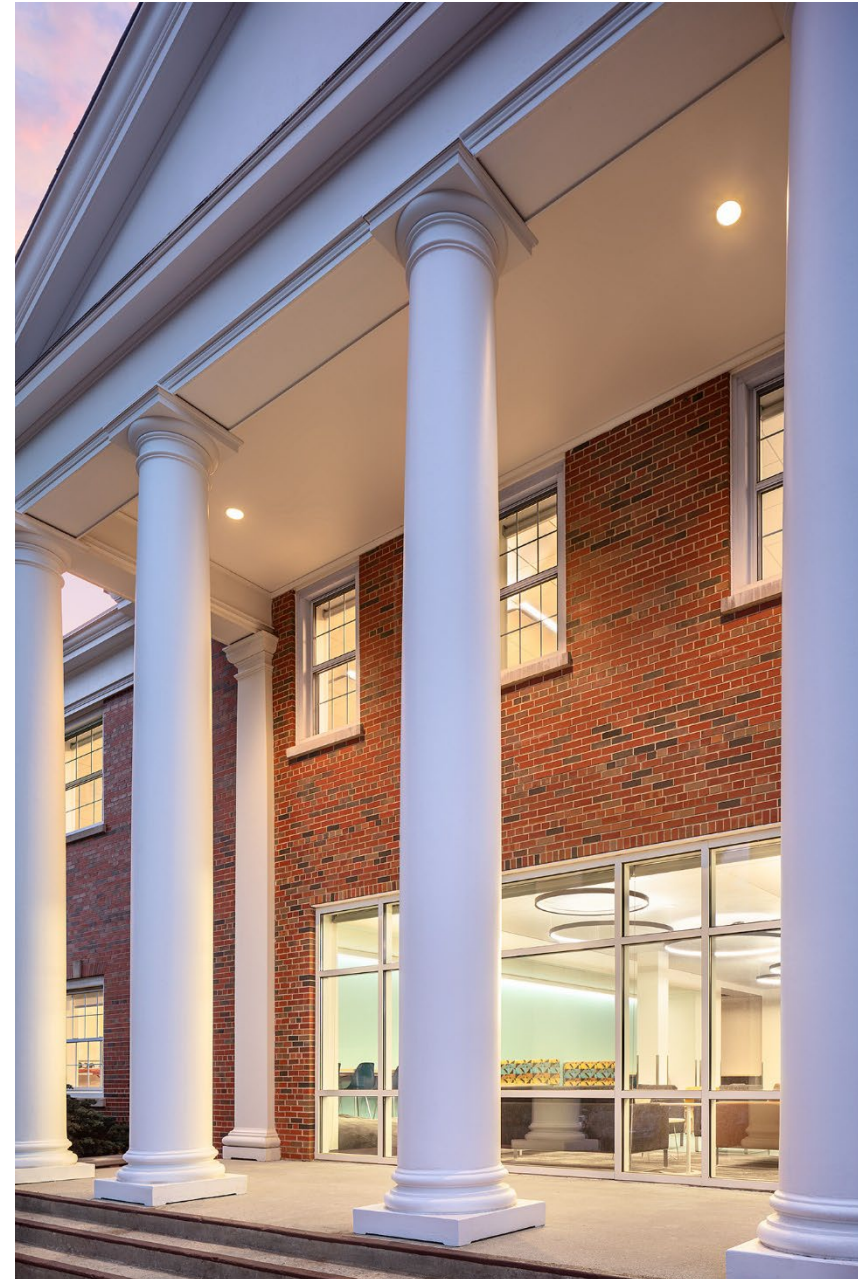
Exterior South Porch
