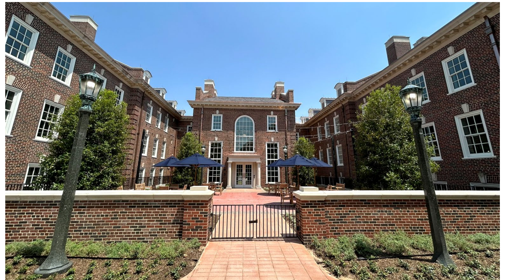
SMITH-PERKINS RENOVATION + EXPANSION
